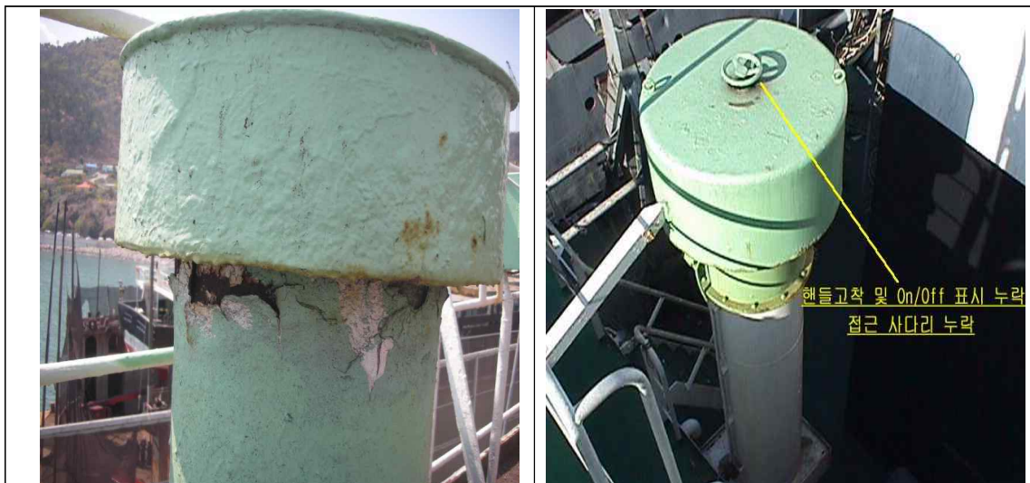
8. Examining the ventilators and air pipes, including their coamings and closing appliances (Ch 2, 202. 1 (6) of the Rules)
